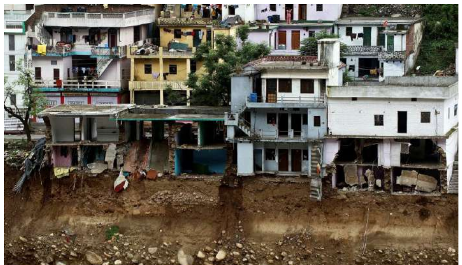
Damaged houses above the flash flood-eroded Mandakini river in the town of Tilwara, around 30km from Rudraprayag, Uttarakhand, in 2013 © Manan Vatsyayana/AFP via Getty Images
